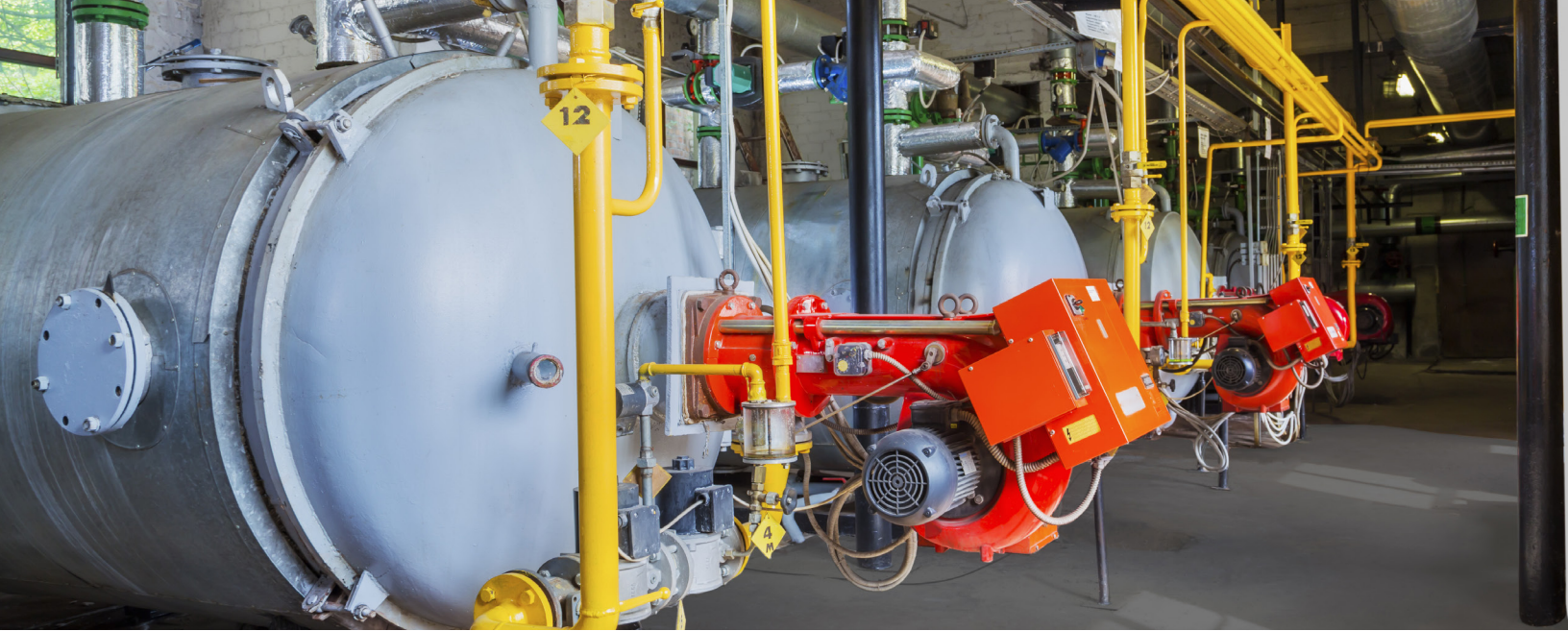
Several natural gas-fired boilers at an industrial facility.
