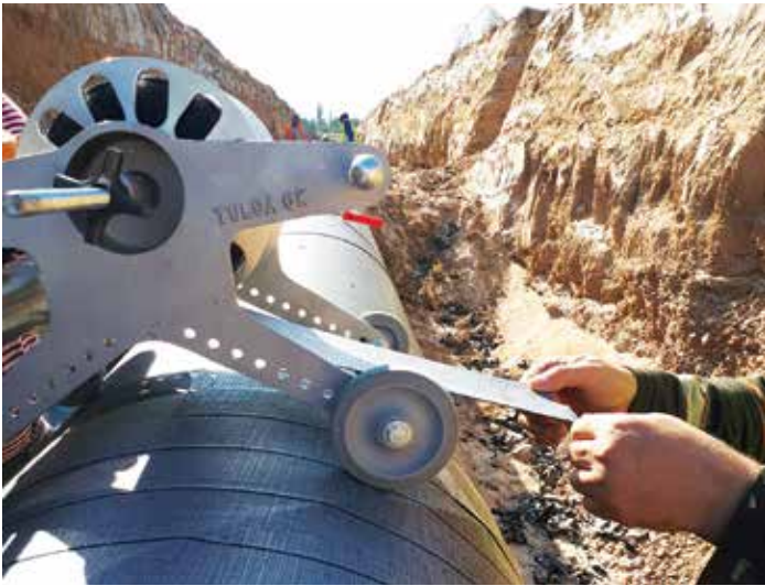
RD-6 quickly bonds to the heated surface and can be permanently adhered.
