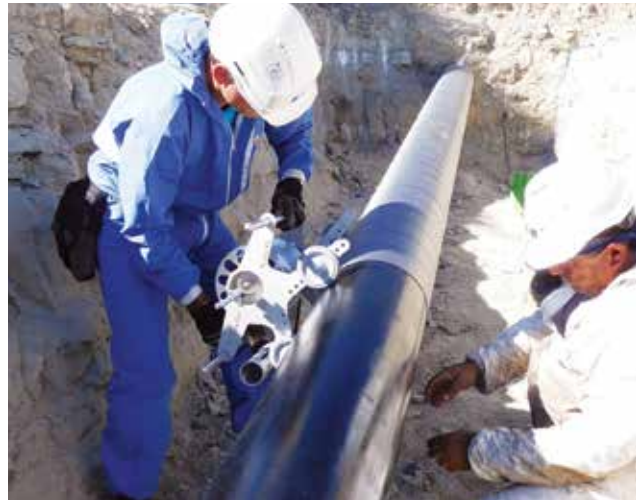
Polyguard Products RD-6 Coating System maintains efficiency in cold weather applications while performing as an excellent non-shielding corrosion coating.
