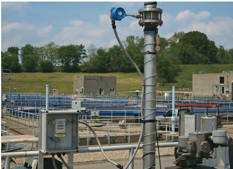
*Here a thermal mass flowmeter is used for off-gas monitoring in a wastewater treatment facility. The instrument's low-flow measurement capability and data-logging software help operators diagnose upset issues to improve process control.*
