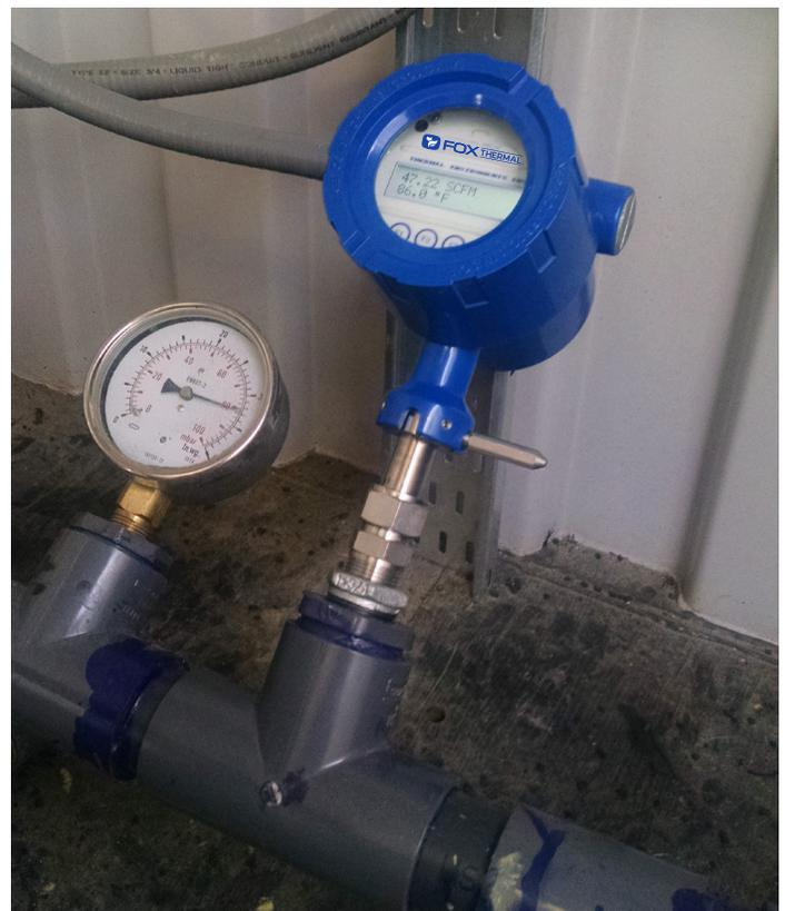
Fox Thermal model FT1 thermal mass flow meter and temperature transmitter.
