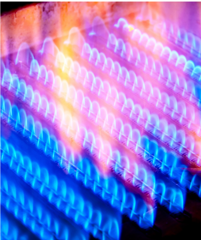
Burner combustion optimization requires the ideal air-to-fuel ratio.
