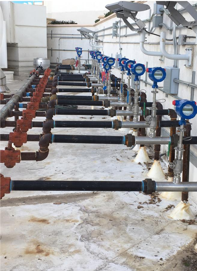
Fox Thermal flow meters used to measure natural gas usage amongst different facilities.
